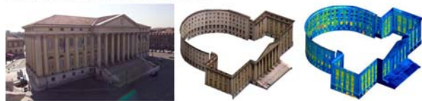
Fig. 7. Palazzo Barbieri in Verona (Italy). Building analysis. Digital reconstruction of a detail from the inner courtyard and the reconstructed 3D model of the exterior walls, visualized with the visible and infrared texture.
